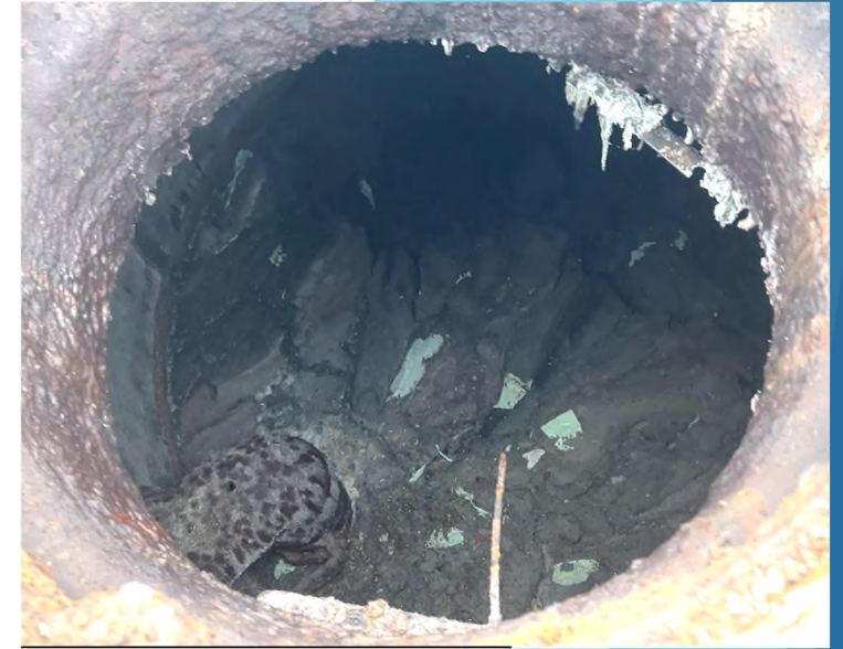
Before IMET Installation - Feb 25 th 2025
