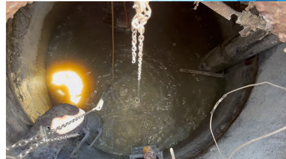
After IMET Installation - June 11 th 2025
